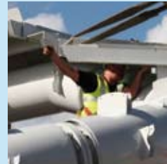
Installation of stair treads and needle being lifted into place
