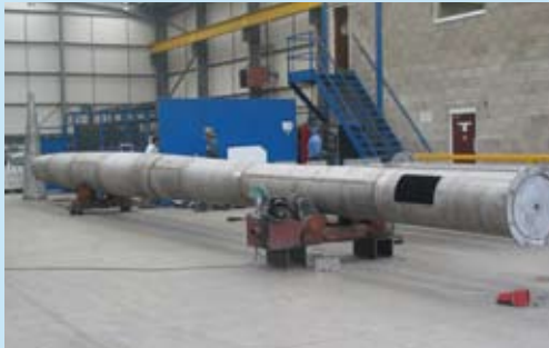
Fabrication of 20-metre stainless steel needle
