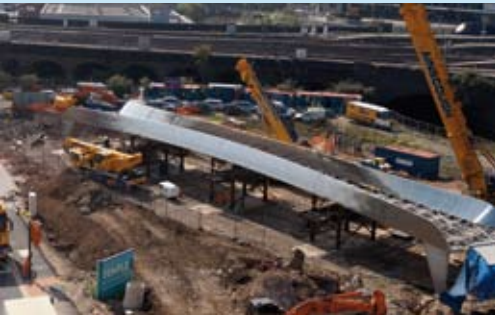
Preparation for bridge installation and bridge lift being undertaken
