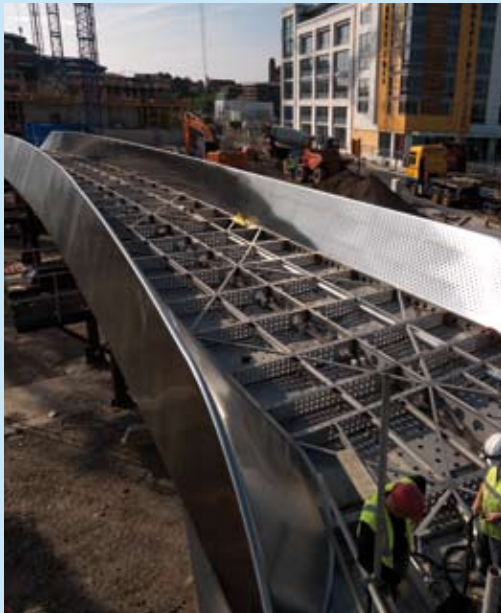
Polishing of welds is inspected
